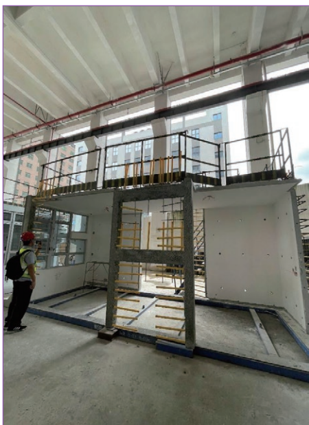
Enhanced edge protection installed at the factory for safer prefabrication and assembly works. 出廠時已安裝強化邊緣防護裝置，以確保預製及組裝作業更安全。
