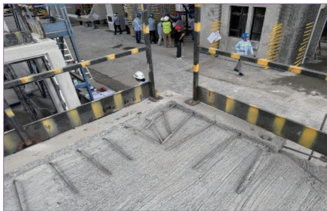
Enhanced edge protection installed at the factory for safer prefabrication and assembly works. 出廠時已安裝強化邊緣防護裝置，以確保預製及組裝作業更安全。
