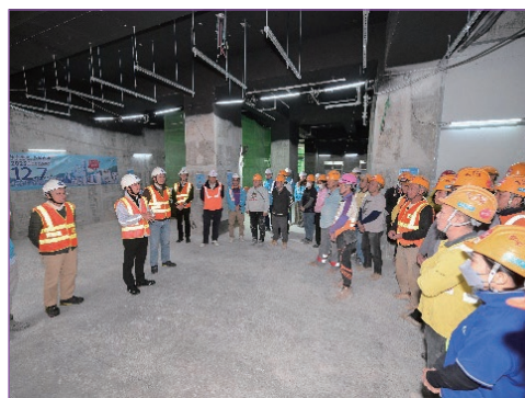
Regular on-site briefings and walkthrough promote hazard awareness and team communication for OHS compliance. 定期進行地盤簡報會與現場巡視，有助提升安全意識及團隊溝通，以確保遵守職安健法規。
