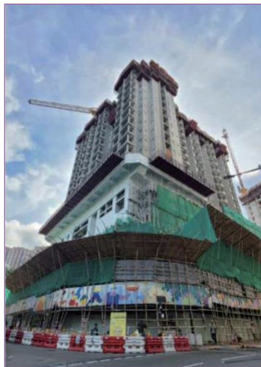
Catch-fan 防護斜棚
